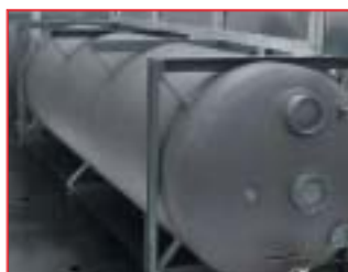
Buffer tank coaxial to the evaporator Wassertank, um den Verdampfer angeordnet
